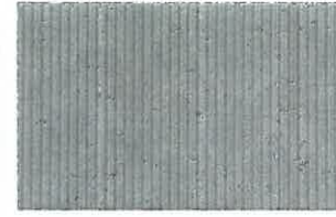
CORRUGATED METAL ROOF
