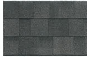
COMP. SHINGLE ROOF
