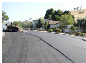
Paving Operation
