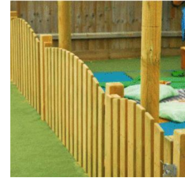
Fence Type 6 - Vertical wood with curved top profile Location: Around playground Height: 5 feet Picket Spacing: 3 1/2" Proposed: New construction
