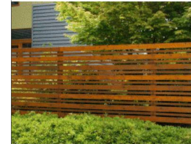
Fence Type 7 - Horizontal wood screen Location: Along Pine Hollow Court Height: 5 feet Proposed: New construction
