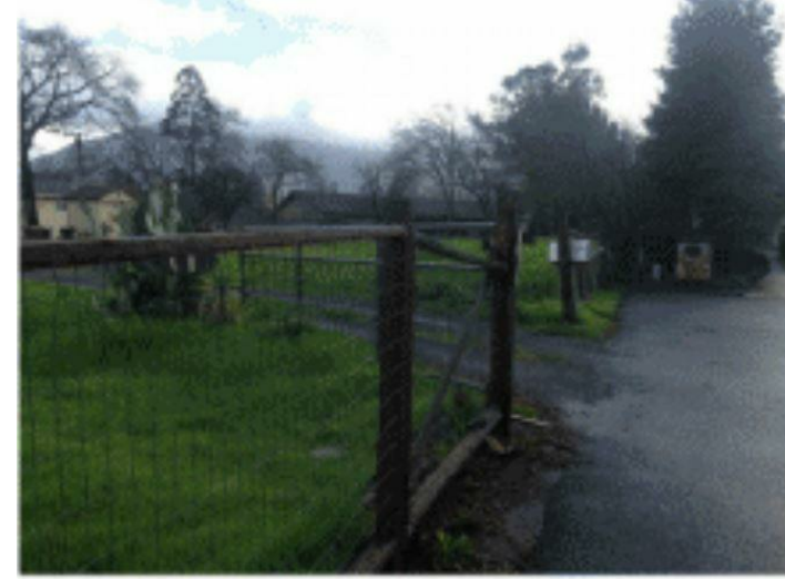
Fence Type 1 - Wood frame and metal screen Location: Along Pine Hollow Court Height: 5 feet Proposed: Demo for new road construction
