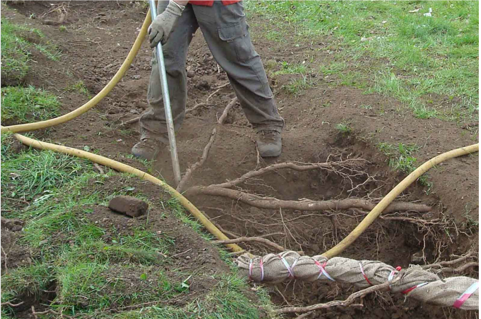
roots exposed by blowing away soil = air spading
