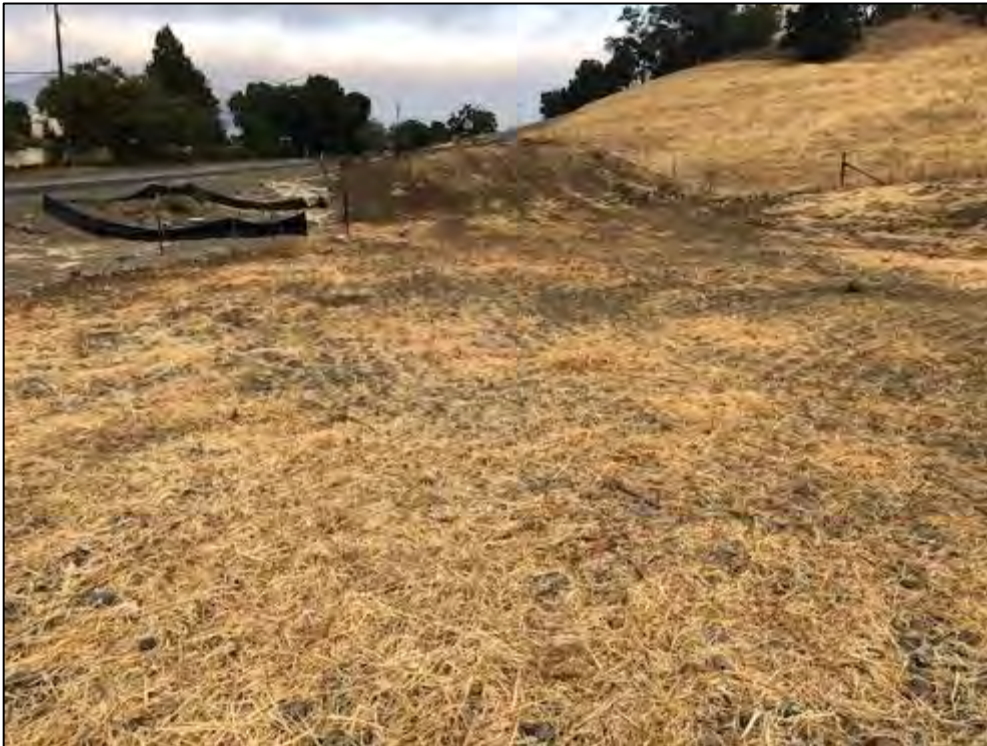
Photo 7. Ephemeral drainage. June 21, 2018. Disced. Culvert to the left with silt fencing.
