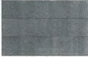
COMP. SHINGLE ROOF
