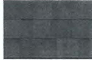
COMP. SHINGLE ROOF
