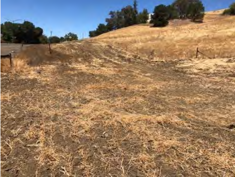
Photo 8. Ephemeral drainage. August 21, 2018. Disced. Culvert to the left with silt fencing.
