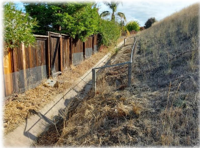
Photograph 24 – Wire fence installed by resident at 1126 Peacock Creek Drive.
