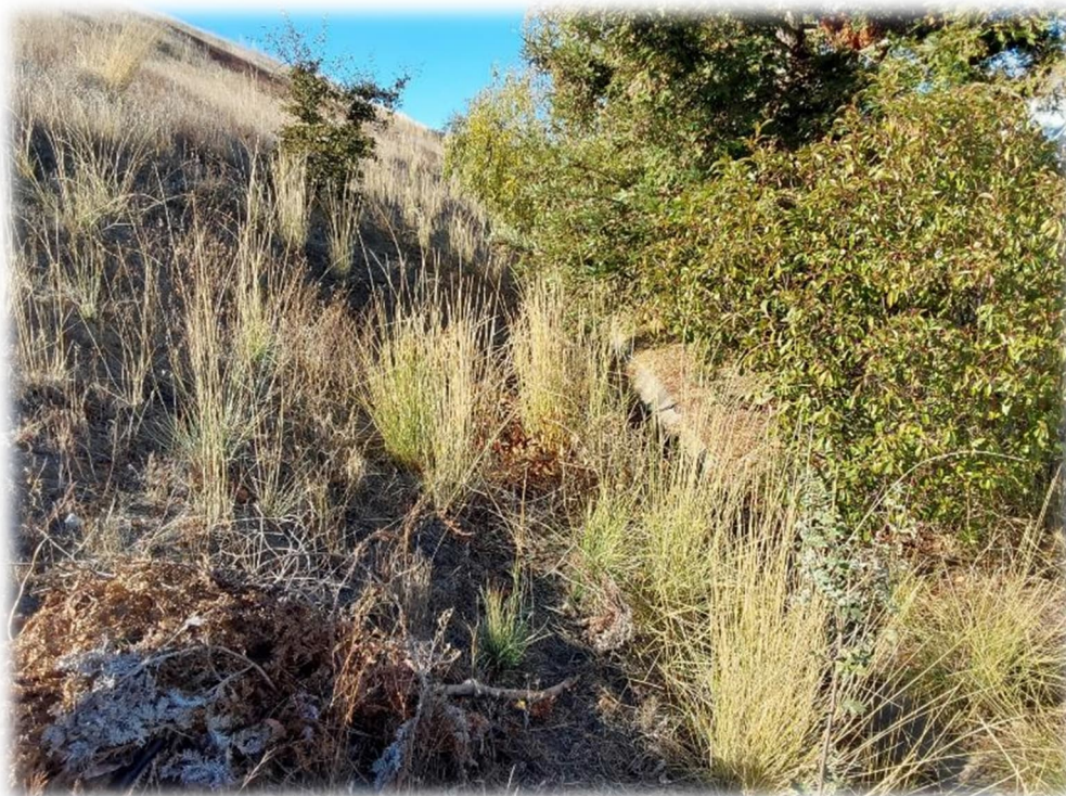
Photograph 14 – Just east of Photograph 12. Additional V-ditch cleaning should be performed.
