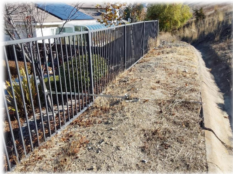
Photograph 11 – Similar conditions observed as noted in March 9, 2023 letter, Photo H: the homeowner has secured trees to the V-ditch beyond property line.
