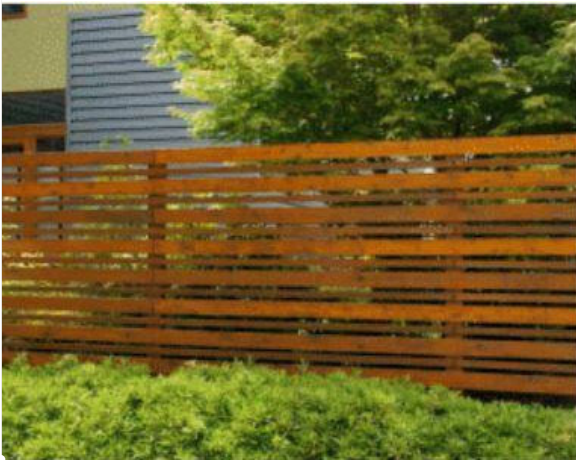
Fence Type 7 - Horizontal wood screen Location: Along Pin Hollow Court Height: 5 feet Proposed: New construction
