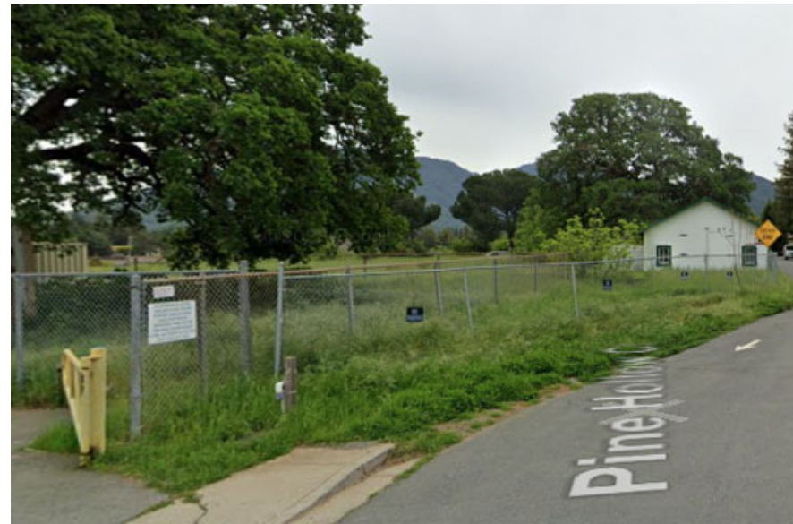
Fence Type 5 - Metal chain link Location: Northwest corner along Pine Hollow Court Height: 6 feet Proposed: Demo for expanded road construction
