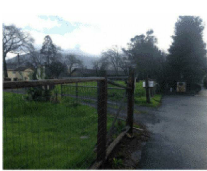
Fence Type 1 - Wood frame and metal Screen Location: Along Pine Hollow Court Height: 5 feet Proposed: Demo for new road construction
