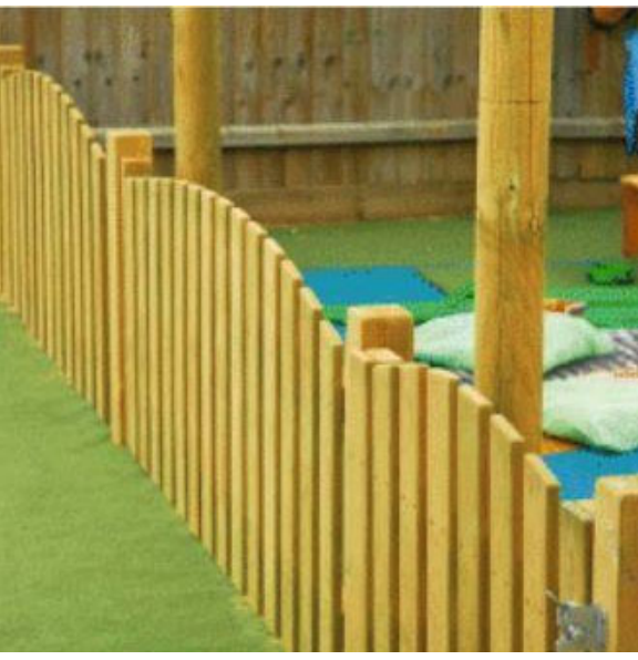
Fence Type 6 - Vertical wood with curved top profile Location: Around playground Height: 5 feet Picket Spacing: 3 1/2" Proposed: New construction
