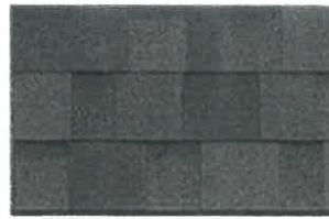
COMP. SHINGLE ROOF
