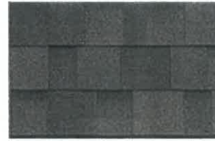
COMP. SHINGLE ROOF
