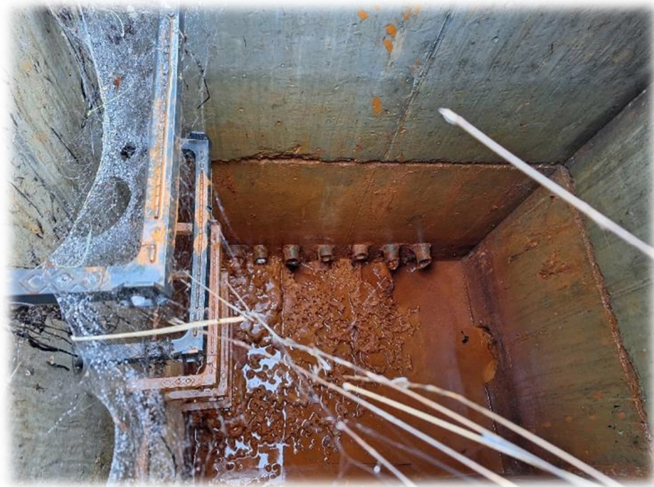
Photograph 8 – Horizontal outlet drain pipes at North Valley Park. Water was discharging from the rightmost pipe only.
