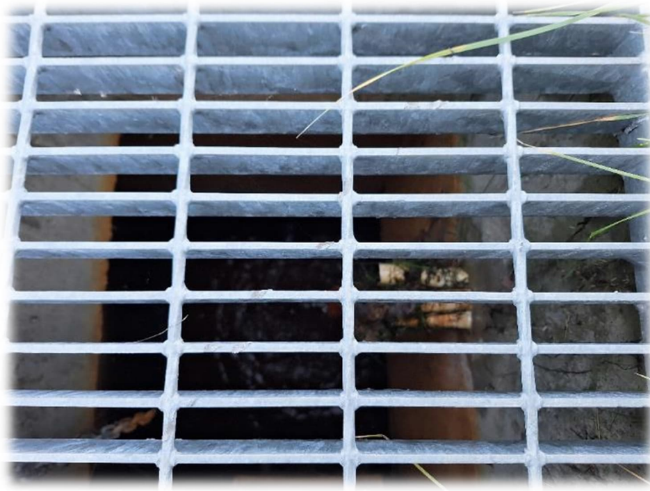
Photograph 7 – Drop inlet at toe of slope at North Valley Park. Pipes are draining but should be cleaned out.
