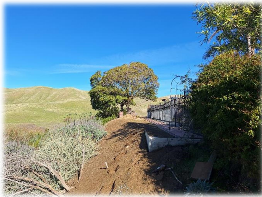
Photograph 10 – Northeastern view of rear of 717 Acorn Drive. Note significant slope disturbance.
