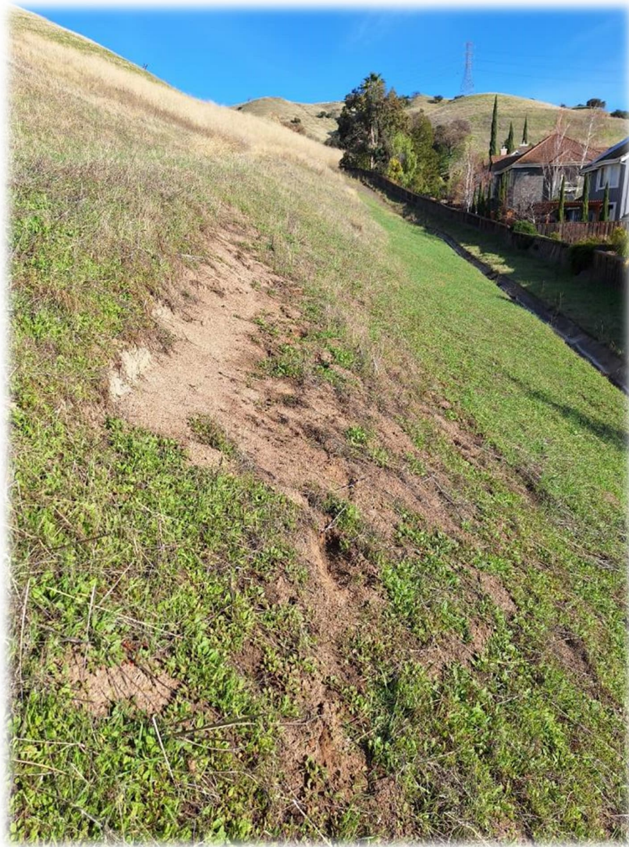
Photograph 4 – Minor slump along slope immediately north of 3061 Windmill Canyon Drive. No movement or bulging observed at toe of slope near V-ditch.
