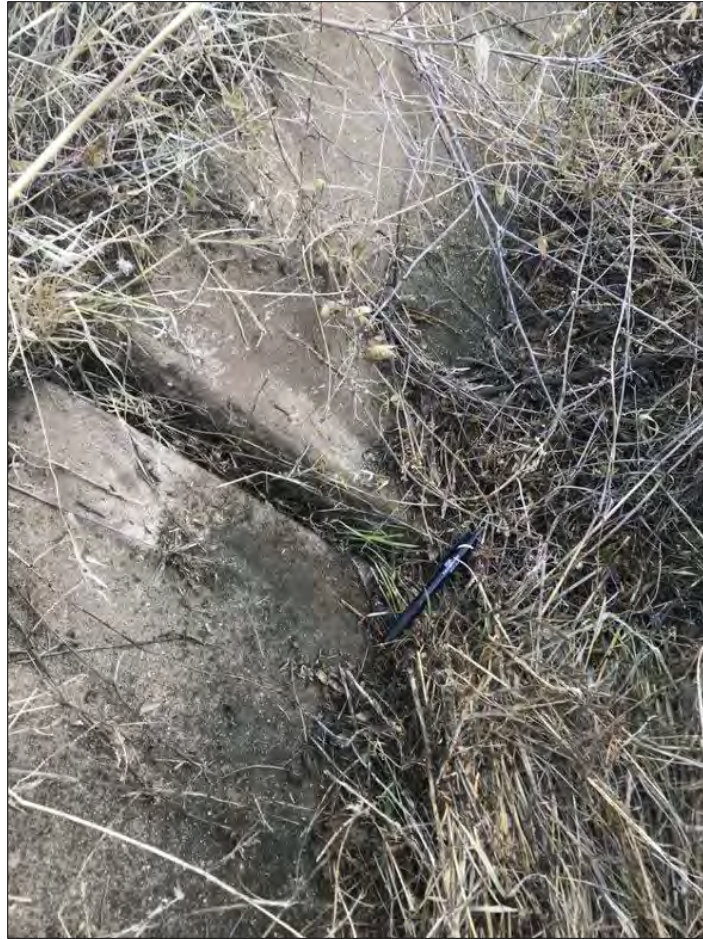
Photo M – Offset and debris in V-ditch northwest of the cul-de-sac at Kelok Way.
