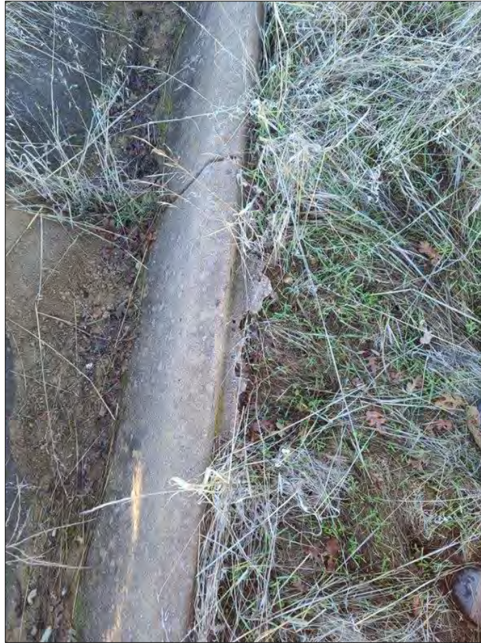
Photo K – Slope creep towards Kelok Way as evidenced by separation of soil from the downhill side of the V-ditch.
