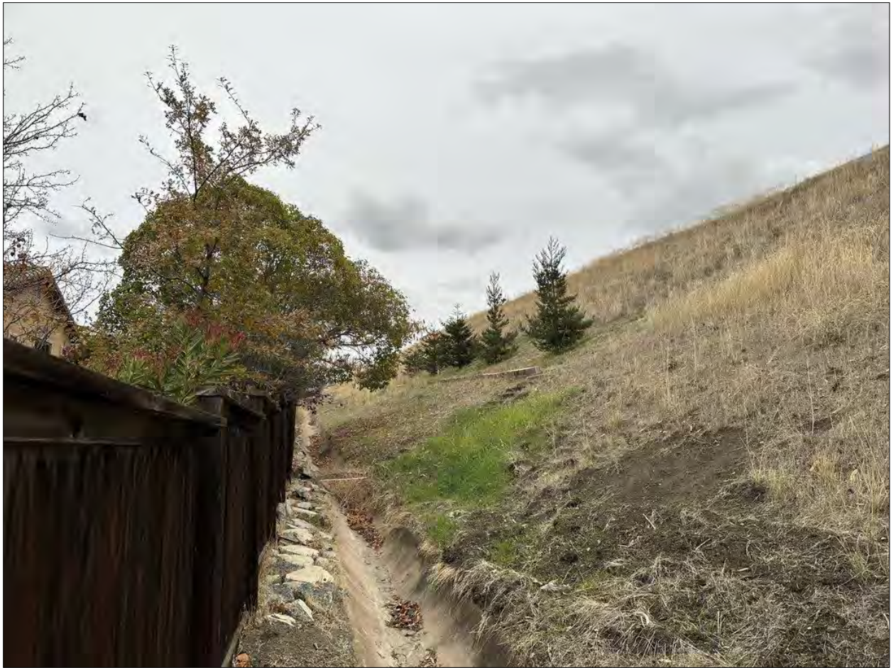
Photo S – Resident has planted trees and built a short keystone-type retaining wall uphill from the V-ditch. Note soil erosion from the disturbed slope sloughing into the ditch.
