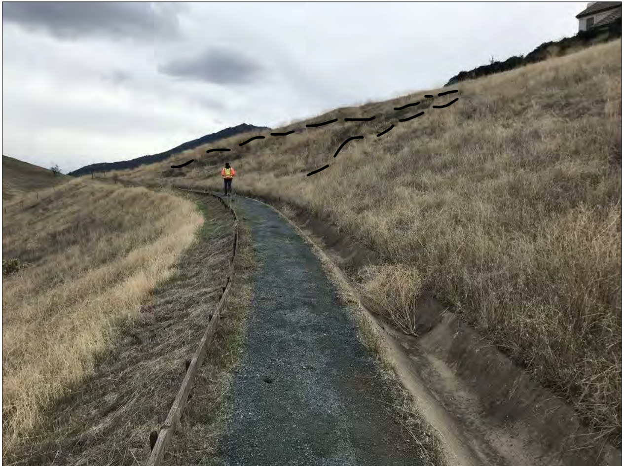
Photo R – Moist slope with shallow sloughing. Note the scarp at the upper end of the movement.
