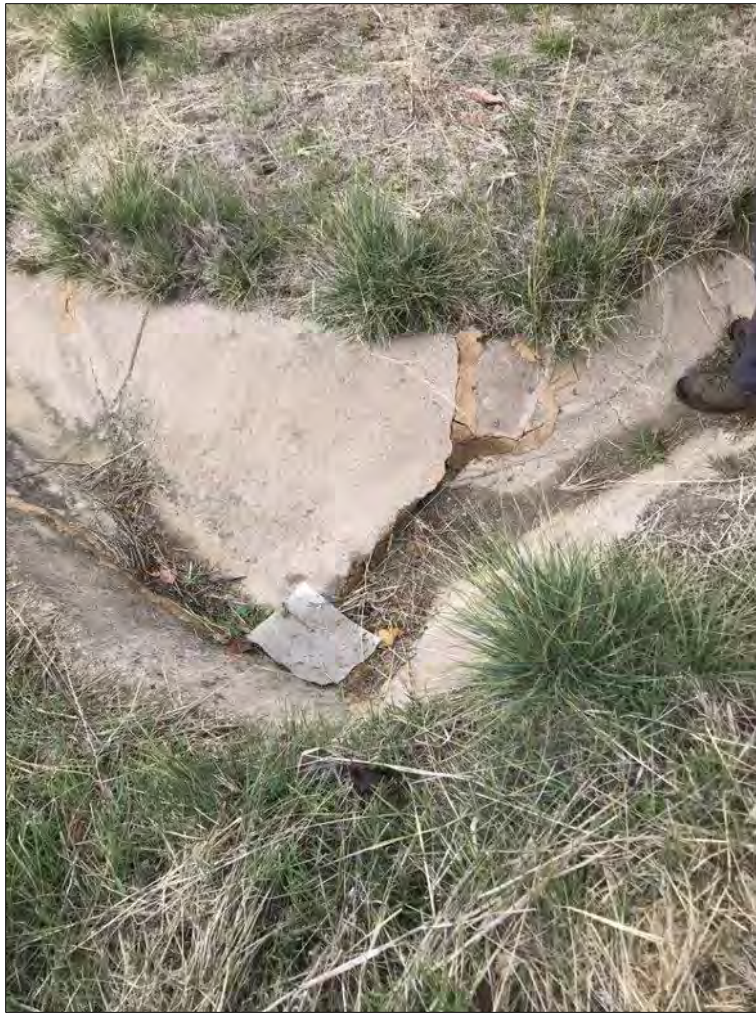
Photo D – V-ditch cracking and displacement East of Windmill Canyon Drive, adjacent to high voltage power line easement.
