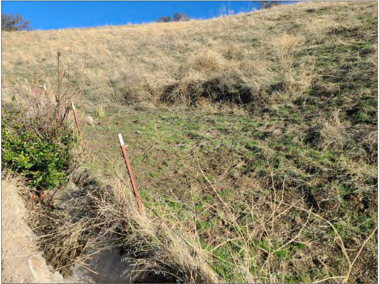
Photo O – Slope creep and minor sloughing adjacent to V-ditch
