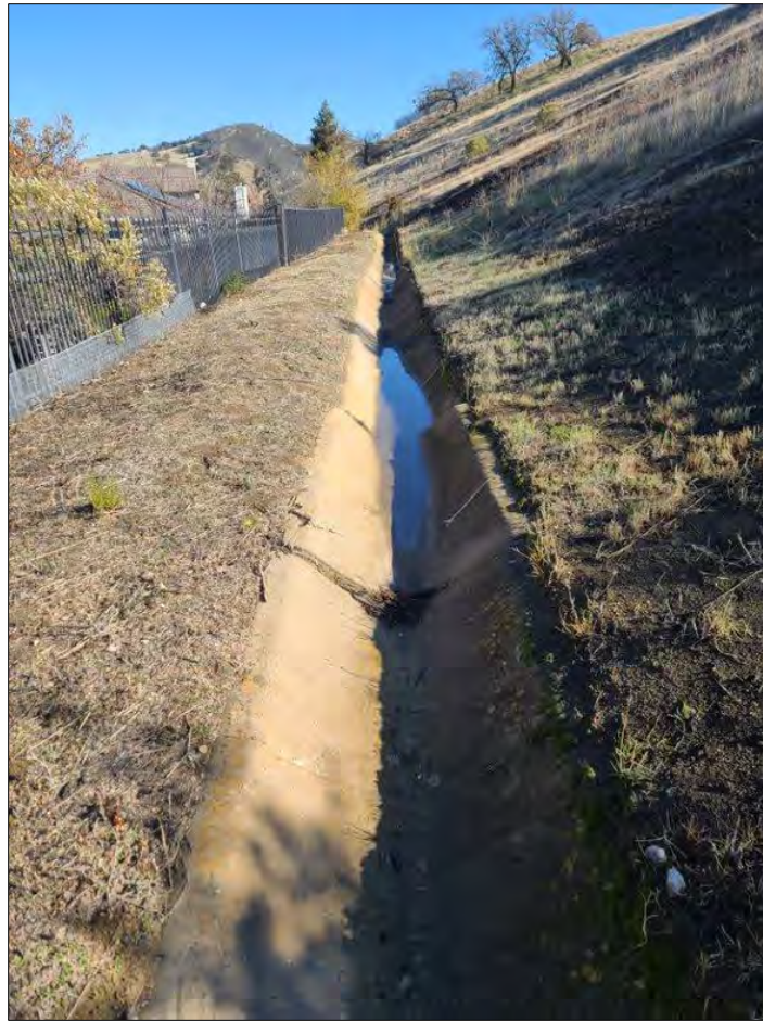
Photo 1 – V-ditch offsets and ponded water. Slope creep is overtopping and possibly offsetting V-ditches.
