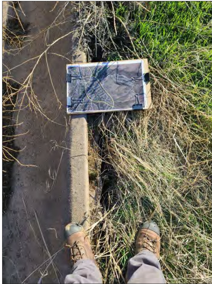
Photo P – Slope creep or expansion cracking adjacent to the edge of the V-ditch.
