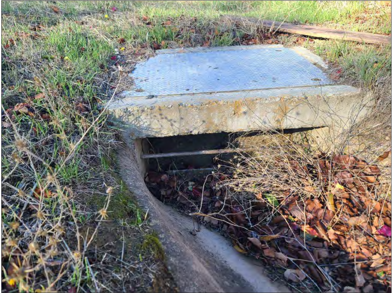
Photo J – Catch basin blocked by soil and debris.
