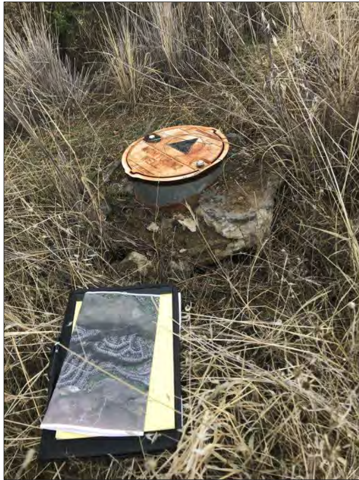
Photo N – Wellhead north (downhill) of the cul-de-sac at Kelok Way. Note that the slope has settled several inches relative to the wellhead.
