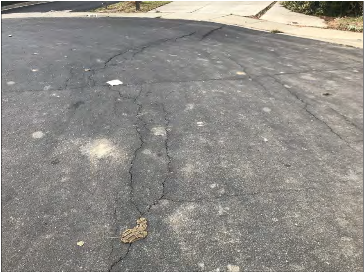
Photo 1 – Settlement/incipient crown scarp impacting the residence (8053 Kelok Way) at the end of the cul-de-sac on Kelok Way.
