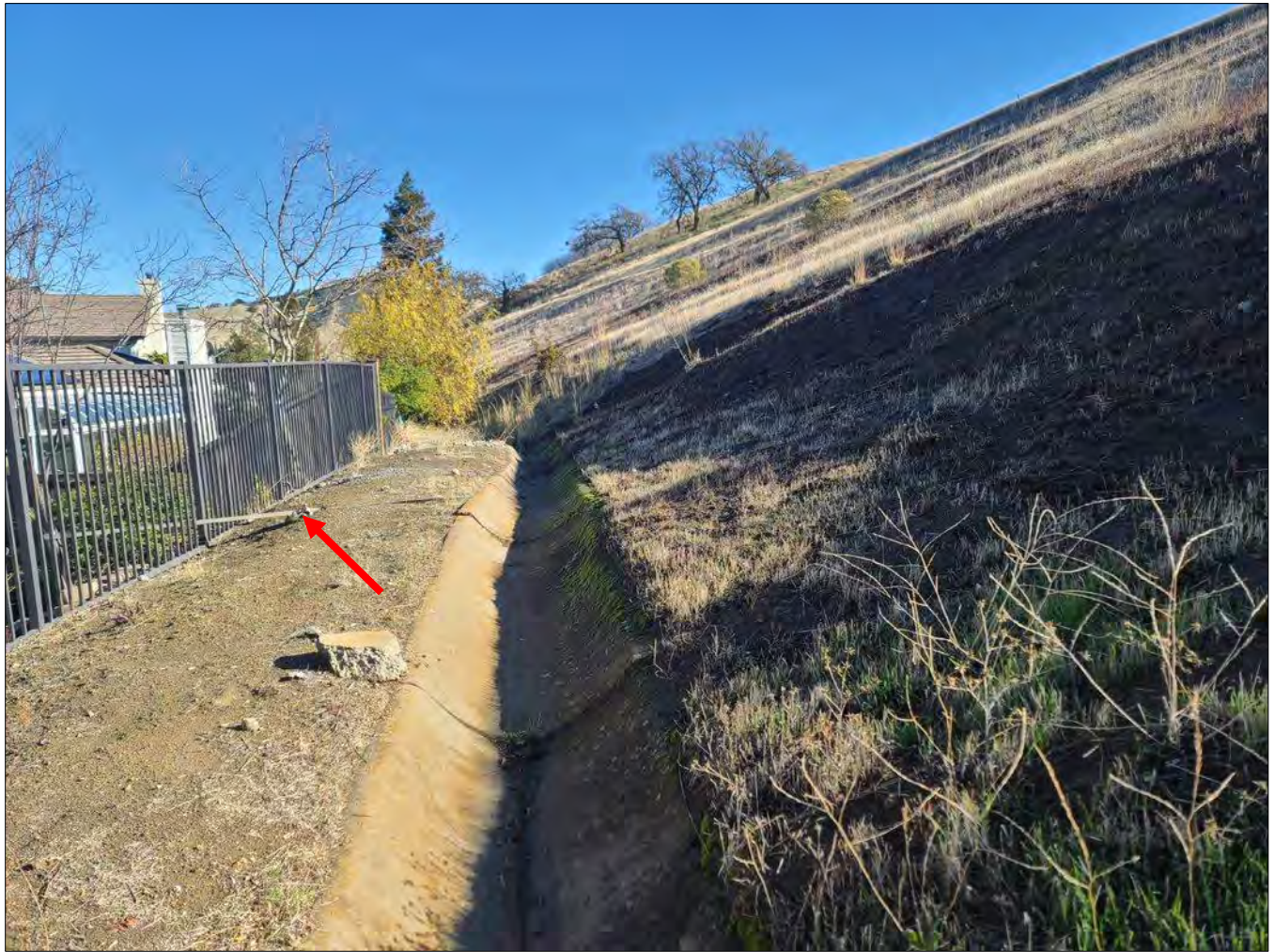
Photo H – Slope creep overtopping edge of V-ditch. V-ditch offsets and shallow raveling uphill visible. Note that the homeowner has secured trees beyond property line (see red arrow), including a V-ditch panel (not depicted in this photo).
