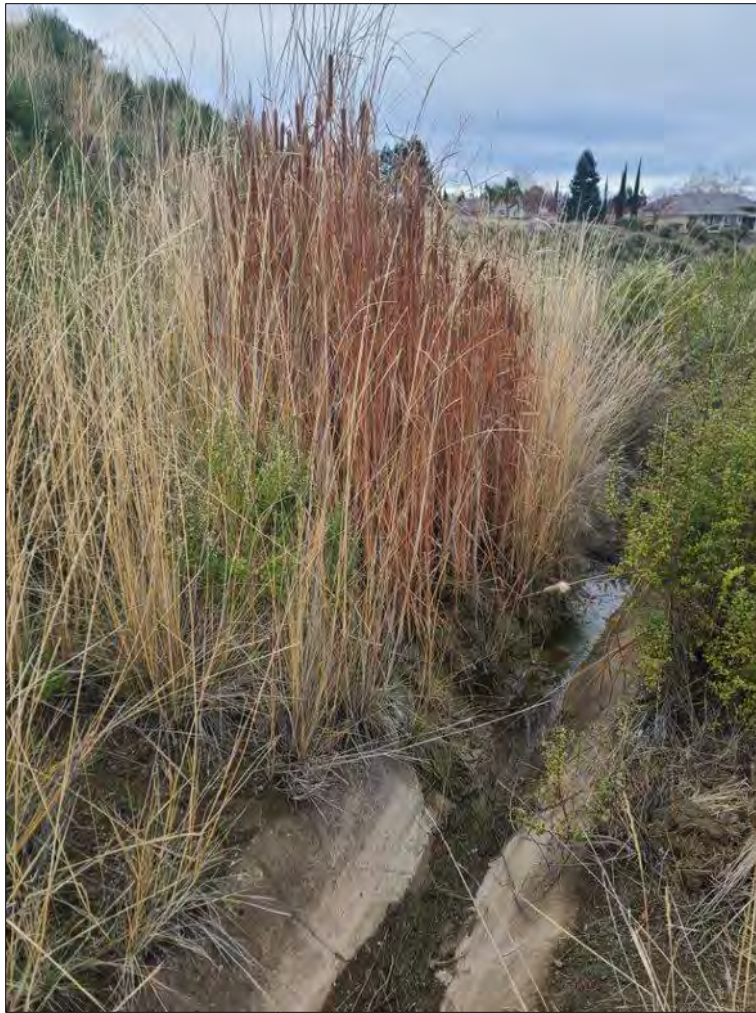
Photo Q – Moist ground and seepage from the slope. Note the marsh grasses and standing water in the ditch.
