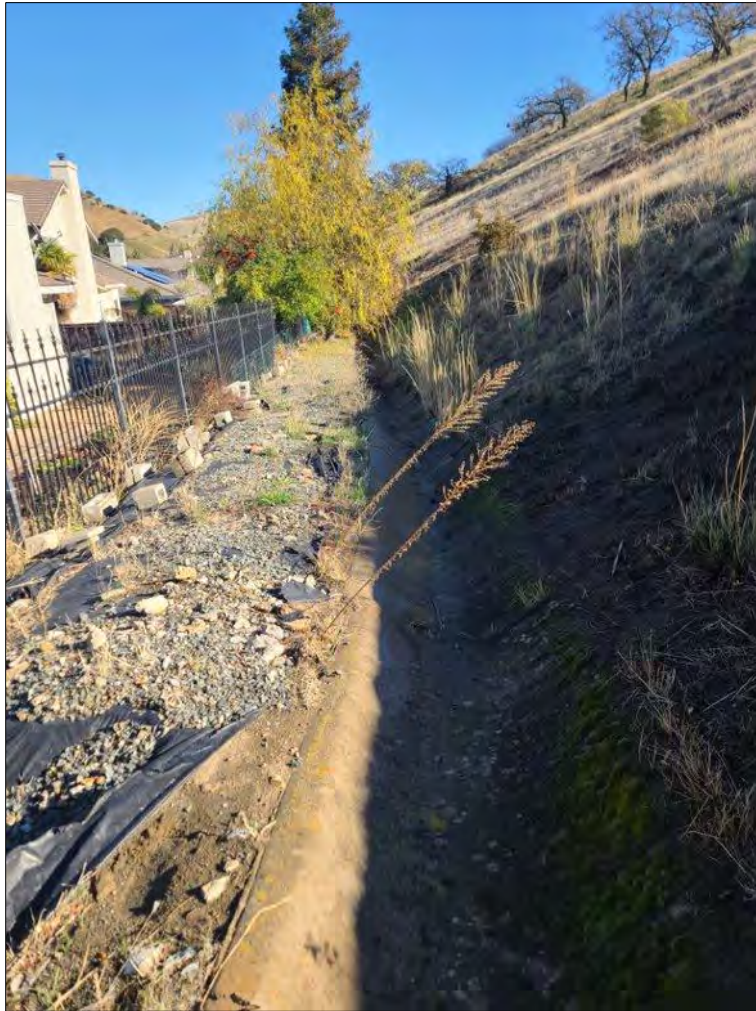
Photo G – Slope creep depositing debris in V-ditch and resulting in minor cracking of V-ditch.
