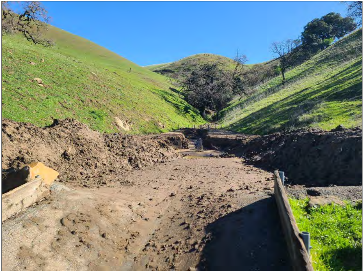
Photo C – Overtopped and eroded debris-flow containment basin above drainage easement northeast of Windmill Canyon Drive. Based on our communication with the City, we understand the erosion and overtopping occurred during the early 2023 rain storms.
