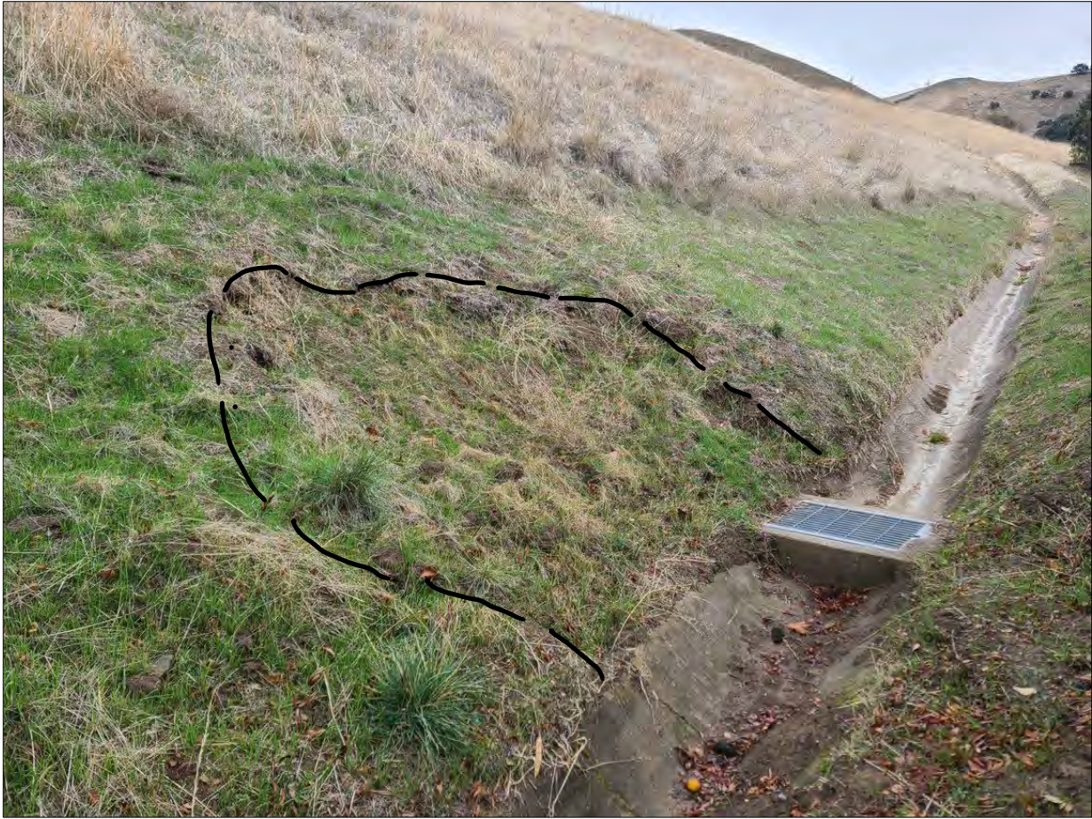
Photo B – Shallow raveling above a drop inlet uphill from Windmill Canyon Drive. Based on our communication with the City, we understand that movement of the uphill from this drop inlet blocked the drop inlet of an uphill V-ditch during the early 2023 rain storms.
