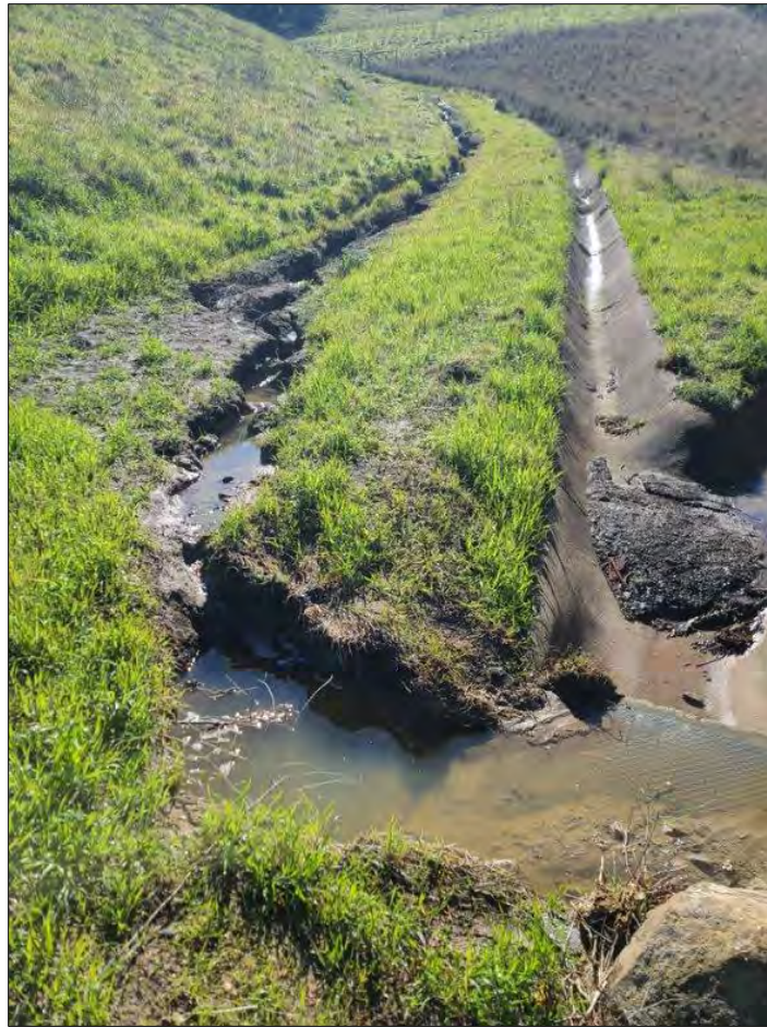
Photo E – Incised gully flow above the V-ditch located East of Windmill Canyon Drive. Erosion and flow occurred during early 2023 storm events.
