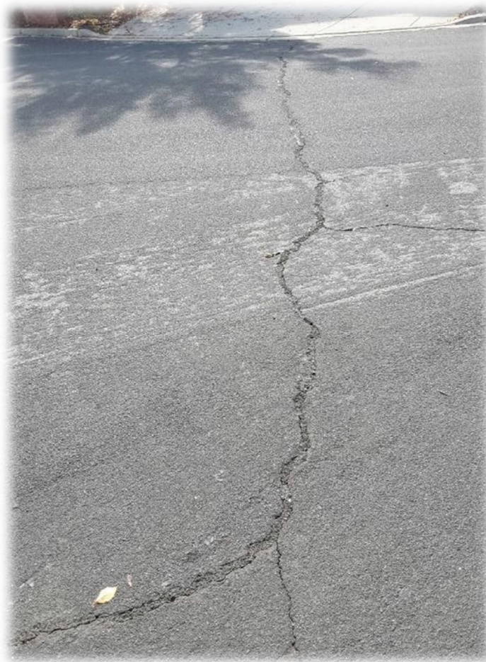
Photograph 33 – Cracks had been filled by City crew within pavement along Torrey Pines as of 11-17-2023.
