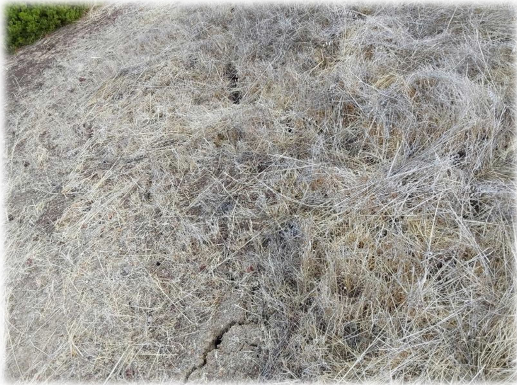
Photograph 17 – Possible slope creep/shrinkage cracks formed along the slope adjacent to/east of Peacock Creek Drive (approximately 40 feet from roadway).
