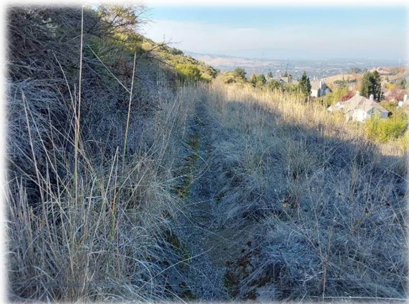
Photograph 8 – V-ditches located along the slope north of Kelok Way contain debris and cracking. Additional V-ditch cleaning and repairs should be performed.
