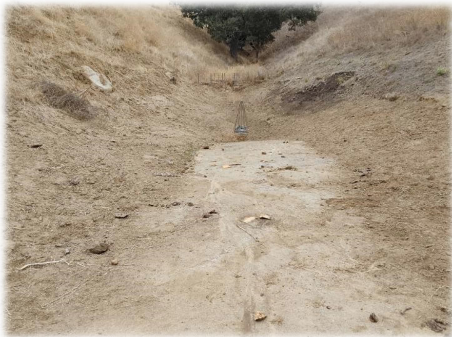
Photograph 4 – Current condition of containment basin northeast of Windmill Canyon Drive. The vertical corrugated metal pipe (CMP) riser contains some soil within it that has accumulated over time. Cleaning of this pipe should be performed.
