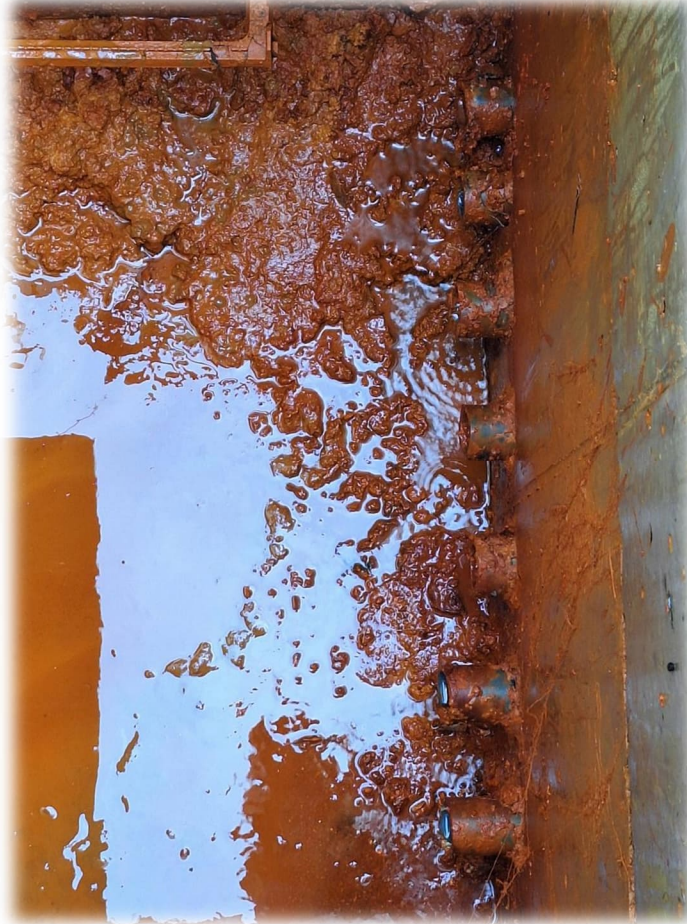
Photograph 16 – Horizontal outlet drain pipes at North Valley Park. Only two of the seven pipes were discharging water on March 5, 2024.
