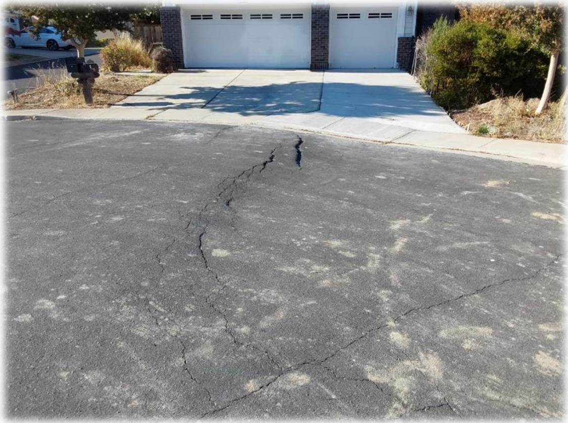
Photograph 5 – Current conditions at 8053 Kelok Way. The cracks have expanded a little and concrete in the driveway/sidewalk has been repaired since we last visited this location (see Photograph 6 below).
