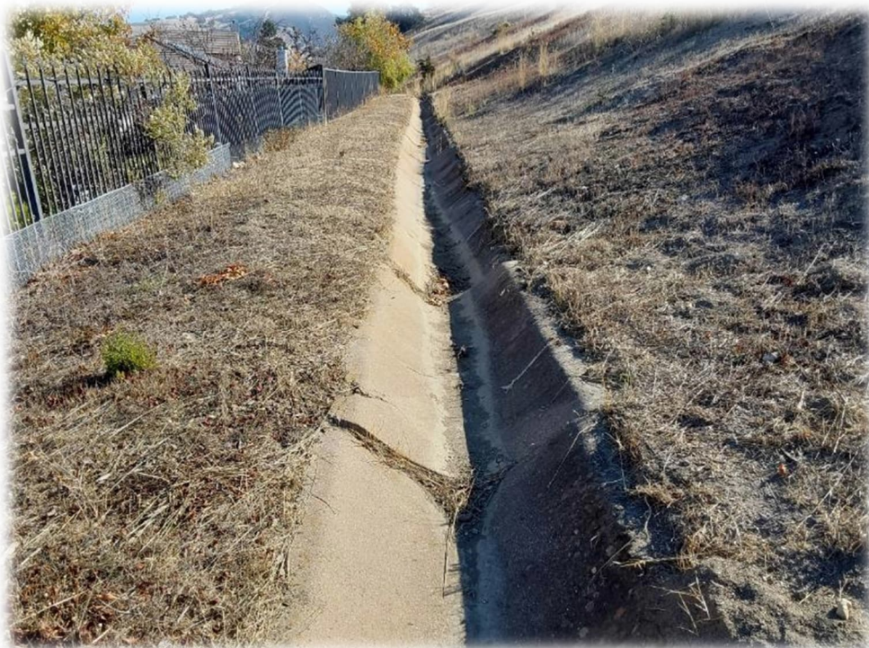
Photograph 10 – ditch condition remains similar as Photo I noted in March 9, 2023 letter: cracked and offset. V-ditch repairs should be performed.
