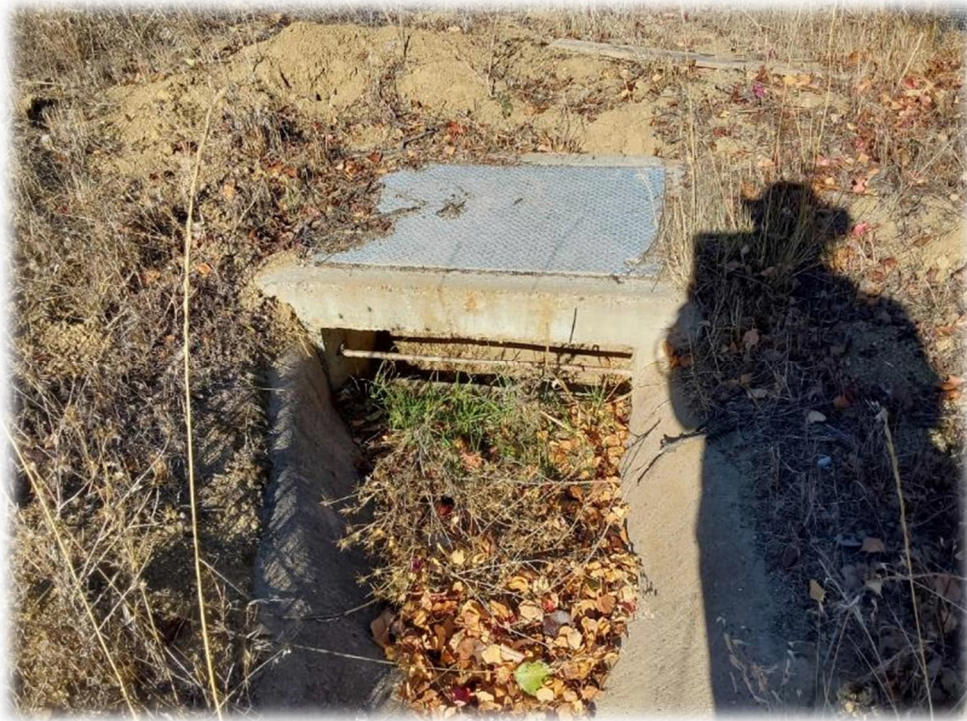
Photograph 9 – Condition of this inlet remains similar to that noted in Photo J of our March 9, 2023 letter: filled with soil/debris. Located west of 8049 Kelok Way. Additional cleaning of this inlet should be performed.
