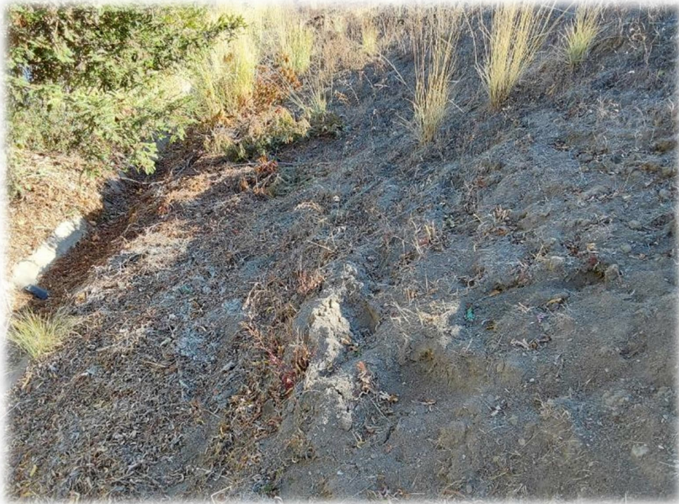
Photograph 13 – Some slope erosion/creep behind 5229 Keller Ridge Drive along with debris within V-ditch. Additional V-ditch cleaning should be performed.
