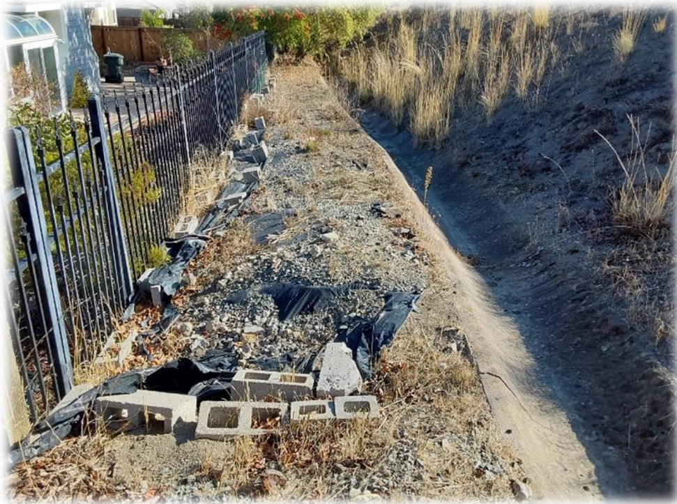
Photograph 12 – Similar conditions observed as noted in March 9, 2023 letter, Photo G: Slope creep depositing debris in V-ditch and resulting in minor cracking of V-ditch. Additional V-ditch cleaning and repairs should be performed.
