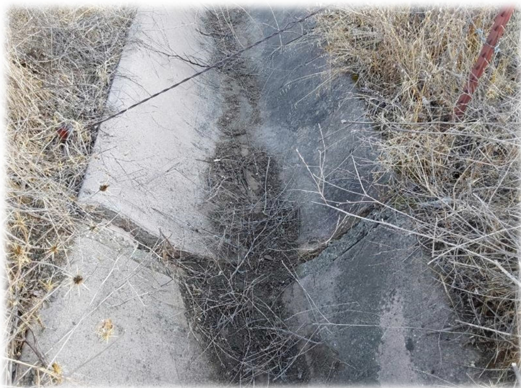
Photograph 21 – V-ditch separated at joint in the area of Photo 18. V-ditch should be repaired.
