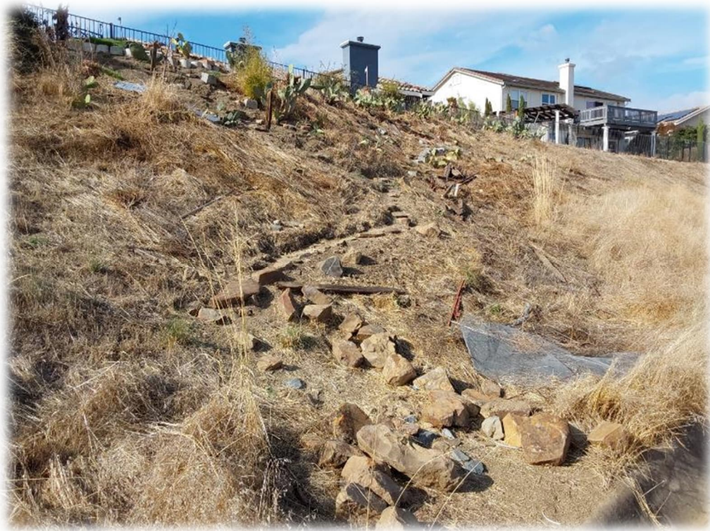
Photograph 28 – Resident at 183 Brandywine Place has added boulders and vegetation to the slope along with creating a pathway, possibly for landscaping purposes. It is not an ideal situation to regrade the slope.
