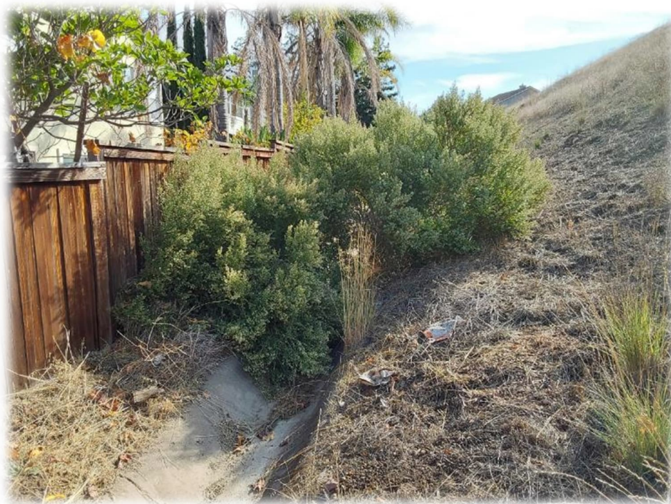
Photograph 26 – Vegetation within V-ditch present just east of Photograph 25 nearly blocks the V-Ditch. Vegetation should be removed from the V-ditch.
