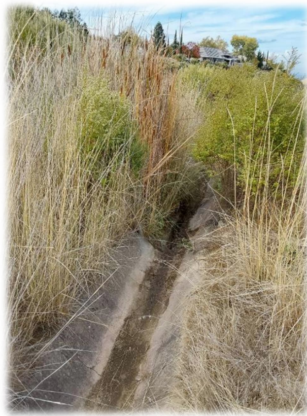
Photograph 34 – Similar conditions observed as noted in March 9, 2023 letter, Photo Q: moist ground and seepage from the slope.
