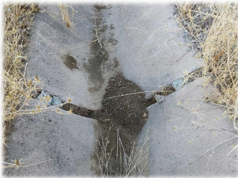
Photograph 20 – V-ditch separated at joint in the area of Photo 19. V-ditch should be repaired.
